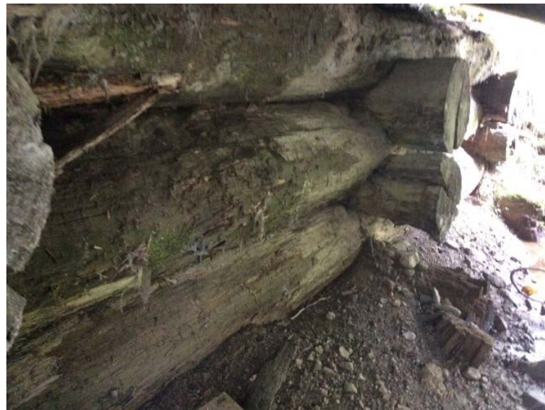
Left Bank Abutment when facing downstream
