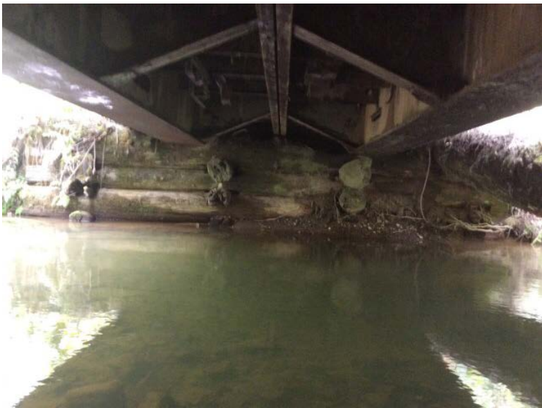
Right Bank Abutment when facing downstream
