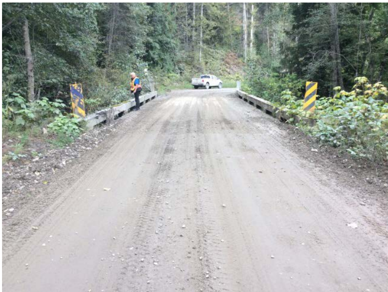
Approach from Right Bank when facing downstream
