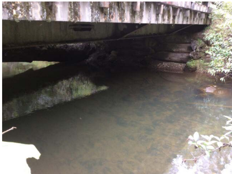
Left Bank Abutment when facing downstream
